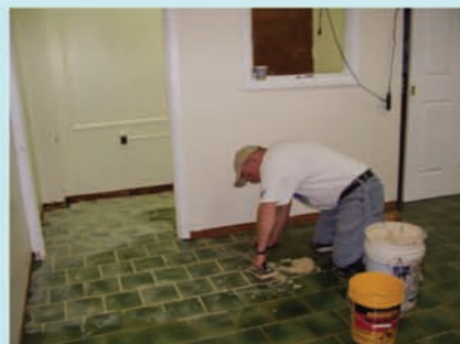
Brian's job is grouting between tiles
