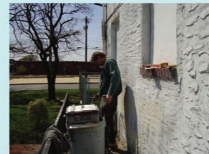
Richard wet-cuts tiles as needed and provides water for cleaning grout from the tiles
