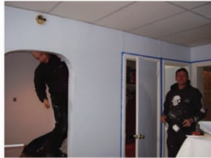
Robert and Richard do final paint touch-ups on second floor
